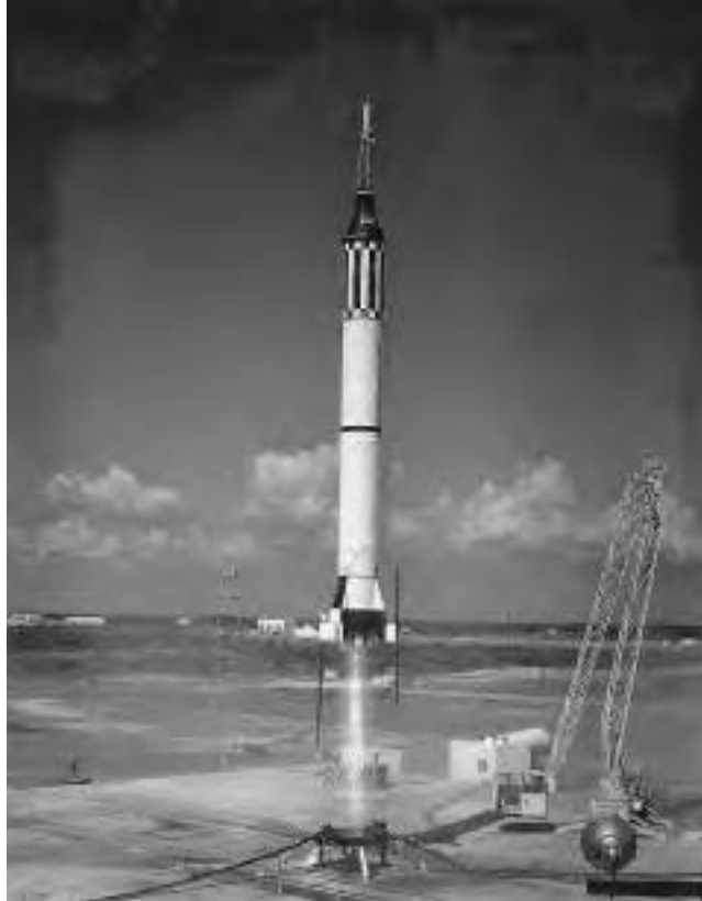
NASA's Mercury Project began with the Mercury Redstone 3 (MR3) mission from Cape Canaveral Air Force Station, Florida, on May 5, 1961. A U.S. Army Redstone rocket successfully carried astronaut Alan B. Shepard, Jr. onboard the Freedom 7 space capsule for a 15-minute suborbital flight, ending with a downrange splashdown and recovery in the Atlantic Ocean. By flying this rocket-propelled ballistic trajectory, Shepard became the first American to travel in outer space. (Courtesy of NASA/JSC)
