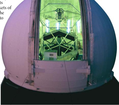
**Domes**, 100 ft (30 m) high, protect the Keck Telescopes. The telescopes themselves weigh 300 tons (270 metric tons) and stand eight stories tall. They are mounted on lightweight frames that provide strength while minimizing weight and cost.
