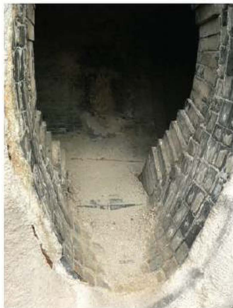
Figure 1.2 A refractory material is one that is physically and chemically stable at high temperatures and is used to line furnaces. Magnesium oxide is a commonly used refractory material due to its high lattice enthalpy.
