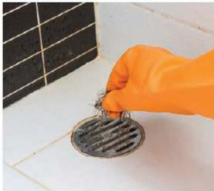
Figure 6.2 Have you ever found hair blocking the plug hole and water pipes? Pouring sodium hydroxide drain cleaner down the drain will help. This strong base will hydrolyse the proteins in hair and help unblock clogged pipes.
