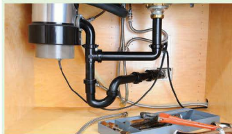
Figure 14.17 These pipes are made from PVC.
