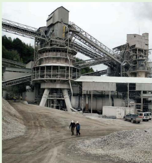
Figure 4.6 A rotary kiln for burning (calcining) limestone into lime, located in Moha, Belgium.
