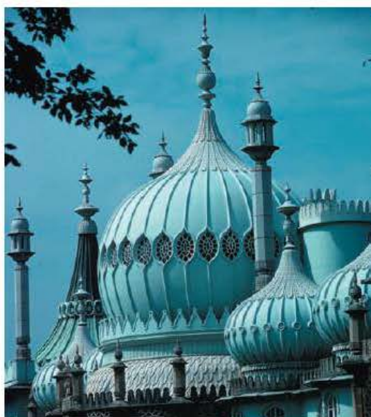
Figure 12.4 The copper dome on Brighton Pavilion is green because the copper has reacted with oxygen in the air to form copper(II) oxide ( \text{CuO} ). This has then reacted very slowly with water and carbon dioxide to form basic copper(II) carbonate, a compound containing both copper(II) hydroxide ( \text{Cu}(\text{OH})_2 ) and copper(II) carbonate ( \text{CuCO}_3 ). Write word equations and then balanced chemical equations for these two reactions.
