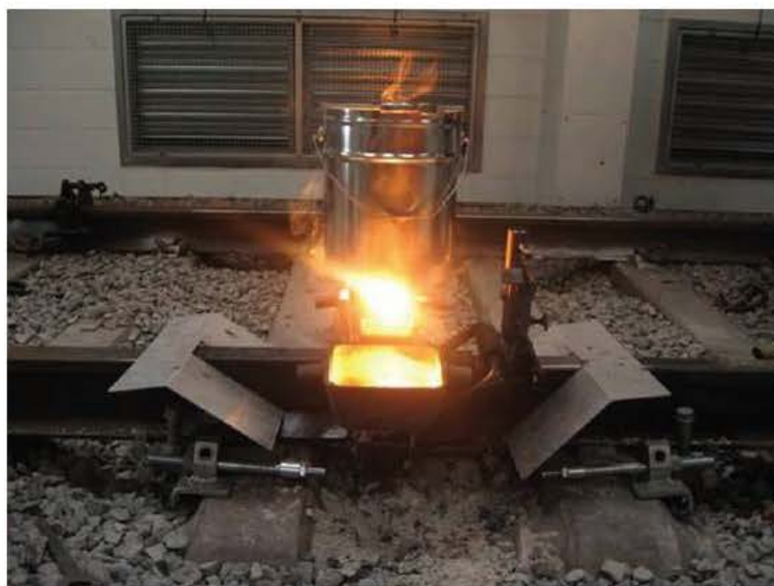
Figure 7.4 The redox reaction between aluminium and iron oxide can be used to weld railway lines together. Molten iron from the reaction runs into a mould around the rails to be joined. When the iron has cooled, the mould is removed and excess metal is trimmed off.
