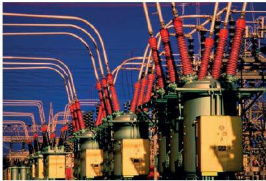
■ Figure 11.37 Step-up transformers at a power station
