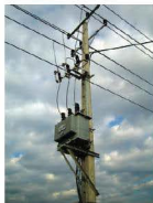
■ Figure 11.34 A transformer on a road-side pole
