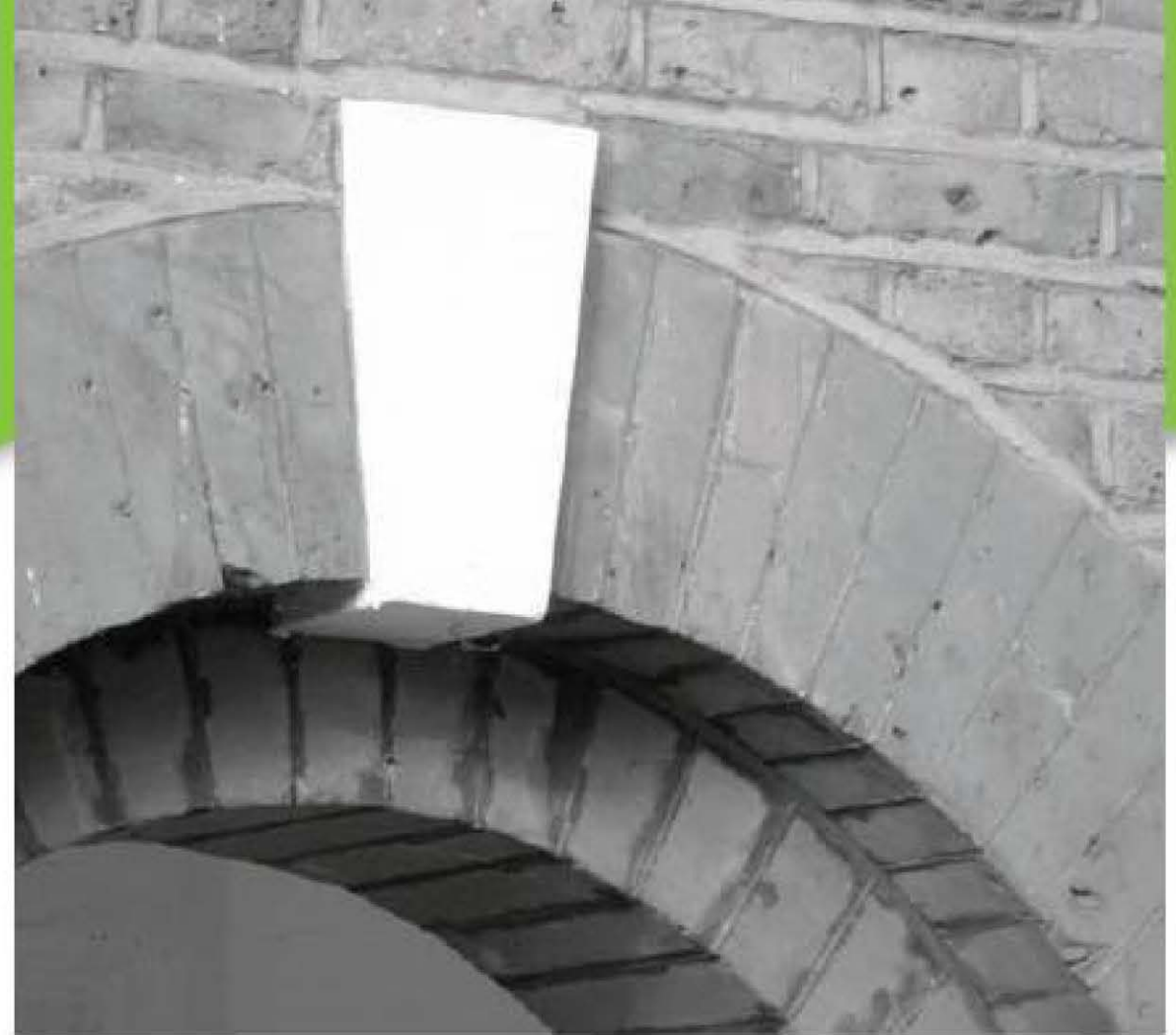
■ Figure 9.25 In architecture, the keystone (shown in white) is necessary to maintain the integrity and shape of an arch
