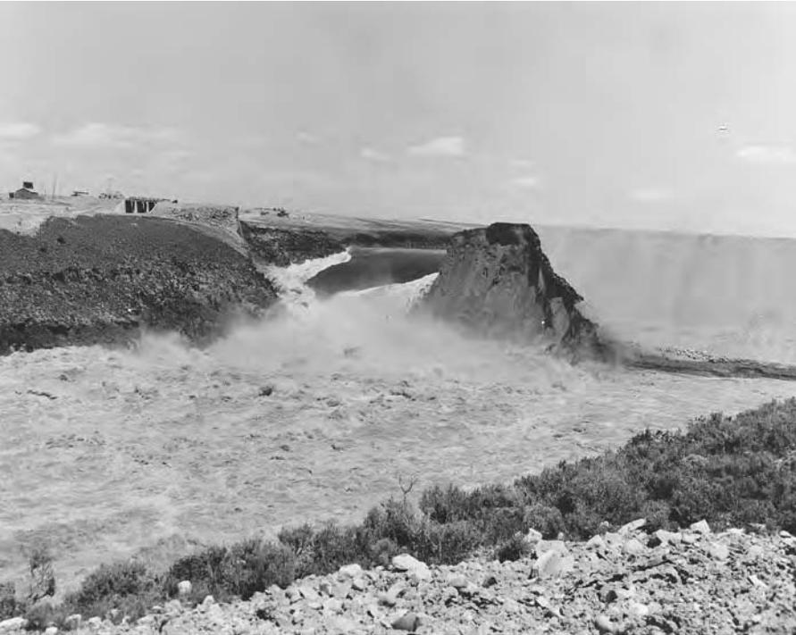
Figure 95 Failure of the Teton Dam.
