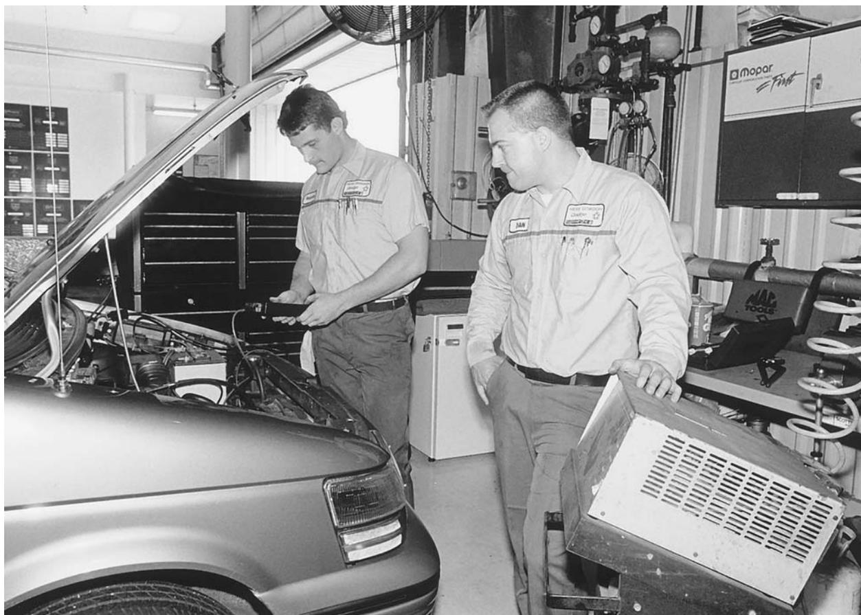
Emissions technicians evaluating automobile emissions in a garage. Technological advances in emissions systems, such as reformulated fuels and catalytic converters, have led to improvements in air quality. (© Martha Tabor/Working Images Photographs.)
