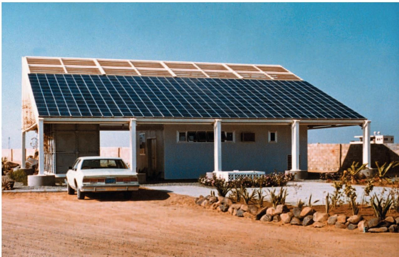
**A custom-designed solar powered desalination system in Jeddah, Saudi Arabia. It is composed of 210 photovoltaic modules that supply 8 kilowatts of power (peak) for conversion of highly saline water into fresh drinking water.** *Mobil Solar Energy Corporation/Phototake NYC. Reproduced by permission.*
