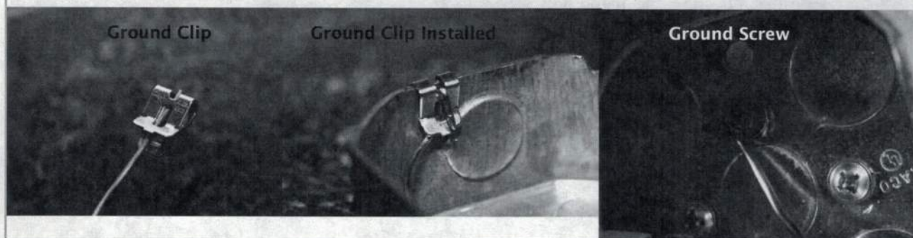
Figure 4-92 Grounding to Frame
