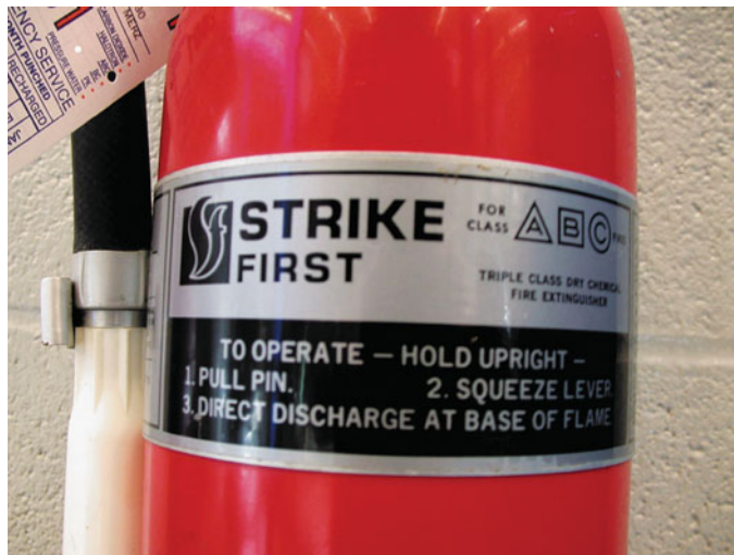
FIGURE 1-79 A typical fire extinguisher designed to be used on Class A, B, or C fires.
