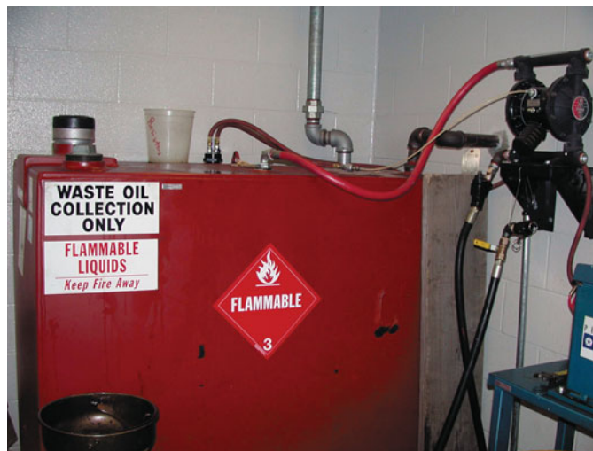
FIGURE 2-3 A typical aboveground oil storage tank.
