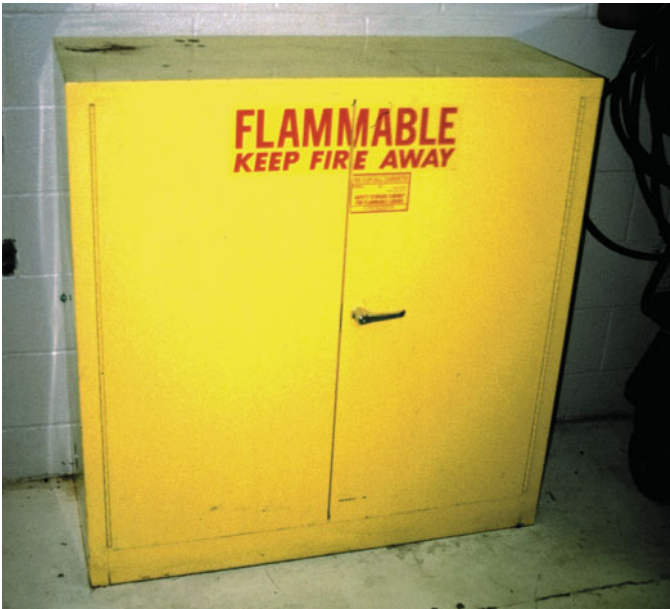
FIGURE 2-5 Typical fireproof flammable storage cabinet.
