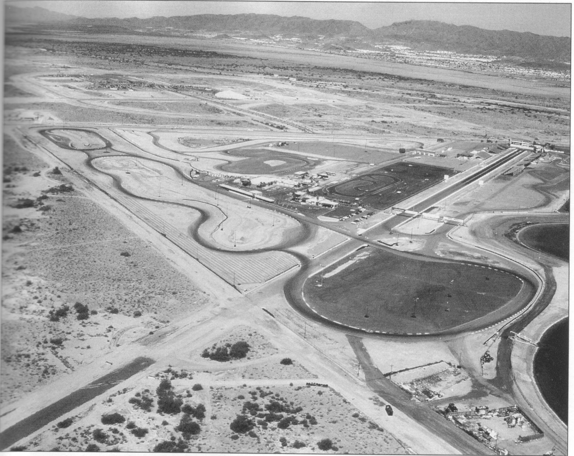
The fastest 60 acres in Phoenix. The Bondurant custom-designed 1.6-mile road course and school facility, Rick Scuteri
