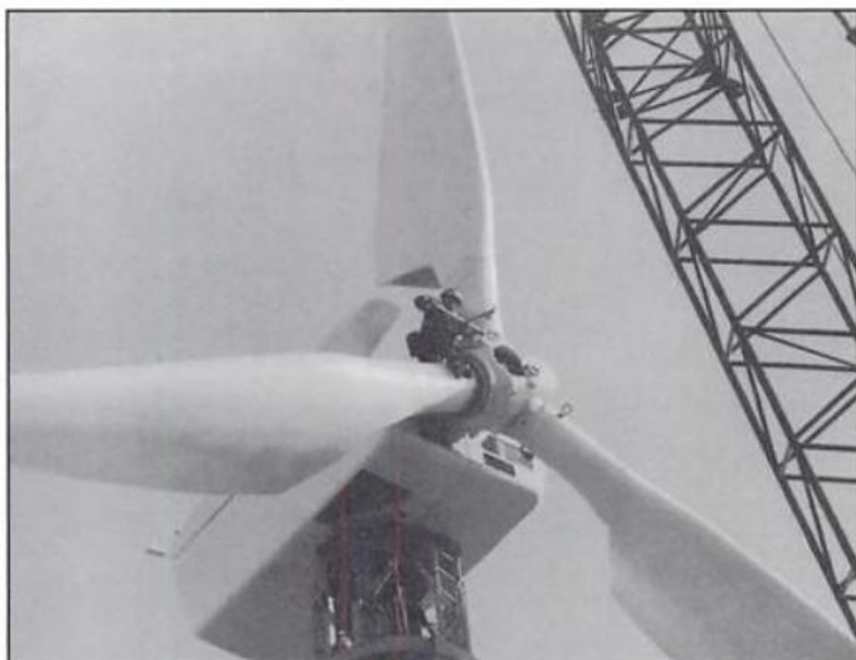
FRP's are also used extensively in the construction of power generating windmills, and for airplane props as well. Photo courtesy Escom Advertising Group, Inc.
