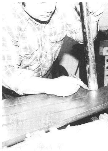
Use a felt-tip marker to indicate where trimming is necessary. Take your time fitting panels.
