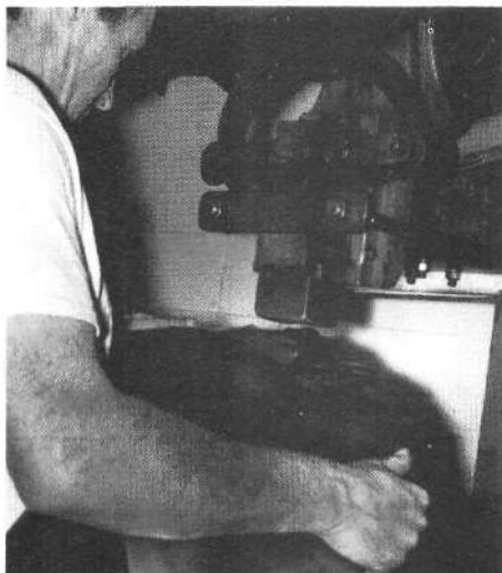
Scott's pulling the first shrinks. He lets the hammer touch the marked line.
