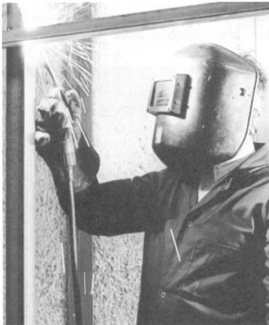
A typical welding situation.
