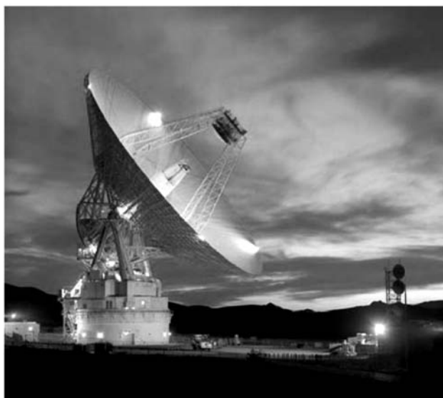
Figure 6. The Deep Space Network (DSN) is an international network of antennae that supports interplanetary spacecraft missions and radio and radar astronomy observations that explore the solar system and the Universe. Via its vital, two-way communications link, the network guides and controls interplanetary explorers and brings back the images and new scientific data that they collect. All DSN antennae are steerable, high-gain, parabolic-reflector antennae.
