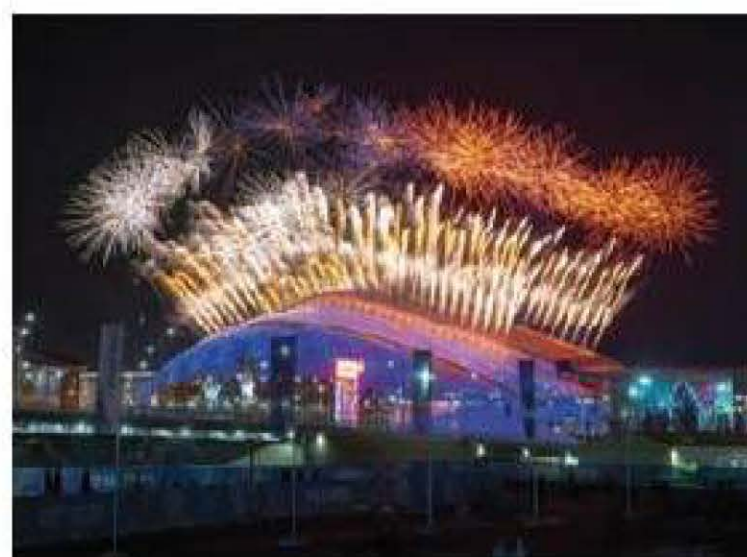
Figure 3.1 Fisht Stadium in Sochi, Russia where the 2014 Winter Olympics were held. The roof is made of a new material called texlon, of which each layer has been engineered to transmit, reflect or scatter the image, enabling the roof to double as a visual display as shown above.
