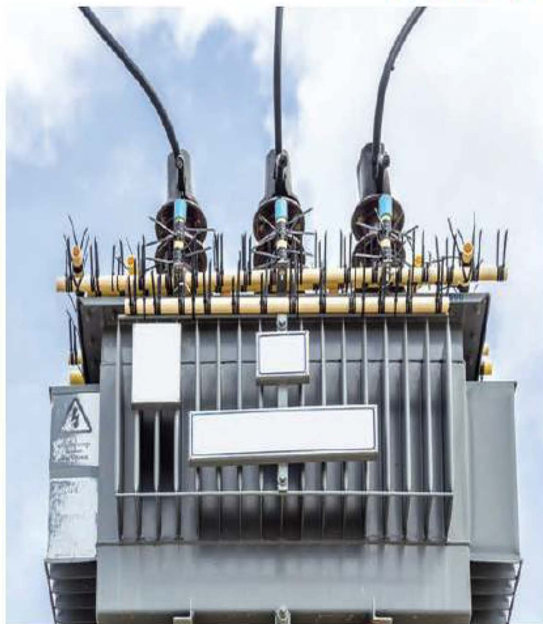
Figure 9.7 Step-up transformers increase the generated voltage from 25 000 V to 400 000 V.
