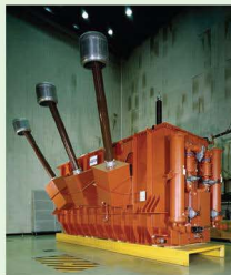
Figure 44.5 Step-up transformers at a power station
