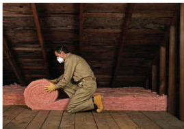
Figure 23.4b Laying lagging in a house loft
