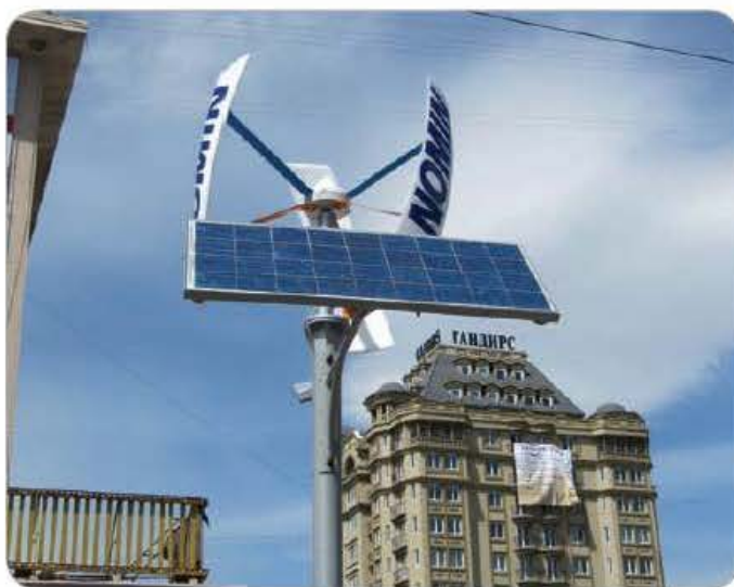
Figure 2.19 Solar panels and mini wind turbines powering street lights in Ulaanbaatar, Mongolia
