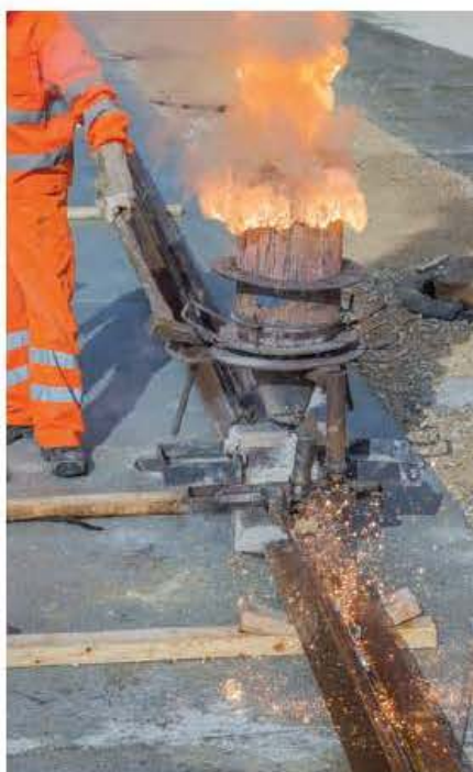
Figure 13.2.16 The thermite reaction between iron(III) oxide and aluminium metal is highly exothermic. The molten iron formed can be used to weld railway lines. The reaction gives out a great deal of energy to its surroundings. The entropy change in the surroundings is large and positive.
