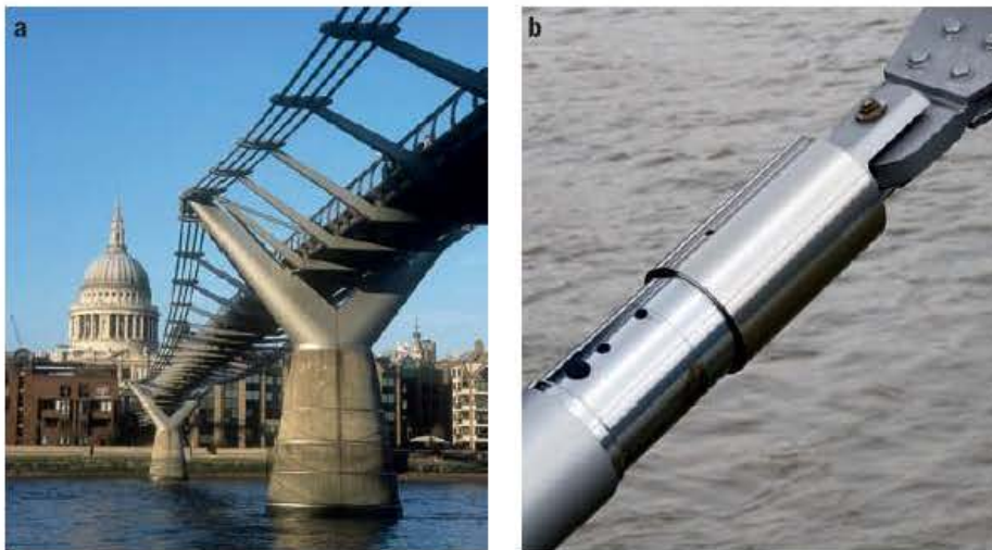
Figure 15.32 a) The Millenium Bridge, London, and b) one of the dampers that had to be fitted
