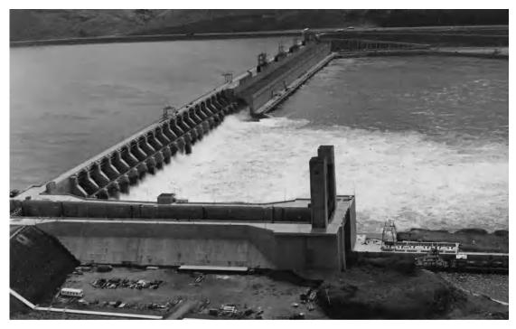
Fig. 1. John Day Lock and Dam, looking upstream across the Columbia River at Washington shore. In the foreground the navigation lock is seen, then the spillway beyond it, and then the powerhouse. The John Day multiple-purpose project has the highest single-lift navigation lock in the United States. (U.S. Army Corps of Engineers)
