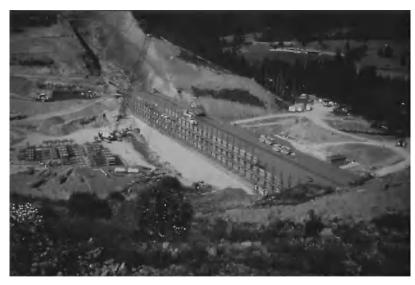
Fig. 13. Galesville Dam, Oregon, showing roller-compacted concrete construction; completed in 1985, it has a height of 157 ft (48 m) and a volume of 161,000 yd<sup>3</sup> (123,100 m<sup>3</sup>).
