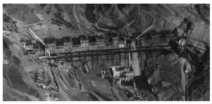
Fig. 9. Block method of construction on a typical concrete gravity dam. (U.S. Army Corps of Engineers)
