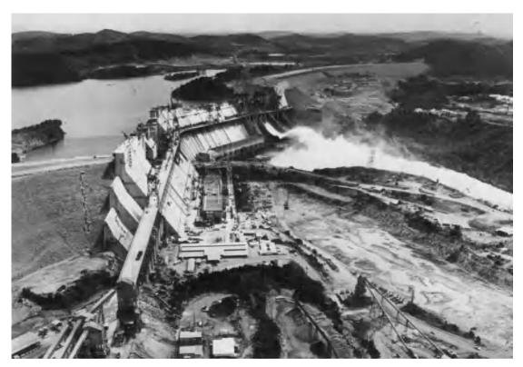
Fig. 3. Guri Dam, Venezuela, showing construction under way on the second stage of the concrete gravity dam. Embankment dams are shown on the left and right abutments. The concrete batch plant is shown at left with a trestle for transporting concrete shown on the downstream face of the dam. The second powerhouse with an excavated outlet channel is shown at the center of the photo. (C.V.G. Electrification del Caroni, C. A. EDELCA, Caracas, Venezuela)
