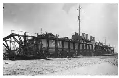
Fig. 2. USS *Delphy* (DD 261), a U.S. Navy World War I destroyer, on a marine railway after being hauled out of the water up the railway at the Boston Navy Yard (since closed) in 1919. (U.S. Navy)
