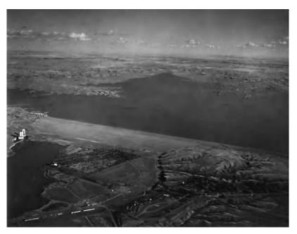
Fig. 12. Fort Peck Dam, Missouri River, Montana, the largest embankment dam by volume in the United States, 125,628,000 yd<sup>3</sup> (95,625,000 m<sup>3</sup>). A hydraulic-fill dam, it was built between 1935 and 1939 for flood control, hydropower, irrigation, and navigation. (*U.S. Army Corps of Engineers*)
