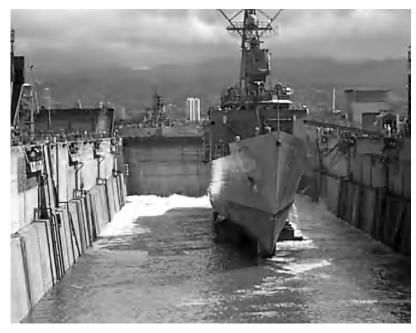
Fig. 6. Graving dock being flooded at Pearl Harbor Naval Shipyard. (U.S. Navy).
