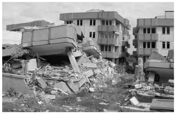
Fig. 1. Relatively new reinforced concrete buildings that collapsed in the Marmara, Turkey, earthquake, August 17, 1999.
