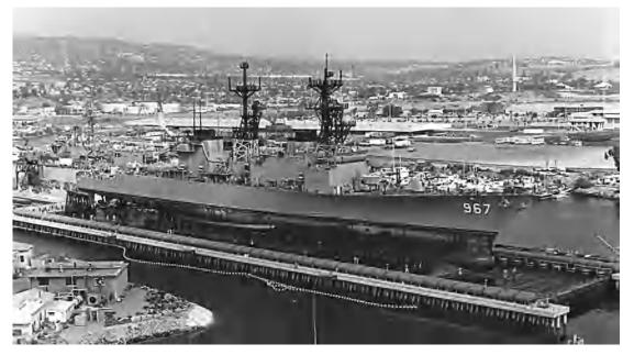
Fig. 7. USS Elliot (DD 967) on a mechanical or vertical lift at the Todd Pacific Shipyard at San Pedro, California, around 1984. When the shipyard closed in the early 1990s, the vertical lift system was disassembled and moved to Malaysia, where it is now operating (as of 2005). (Rolls-Royce Naval Marine Inc.)
