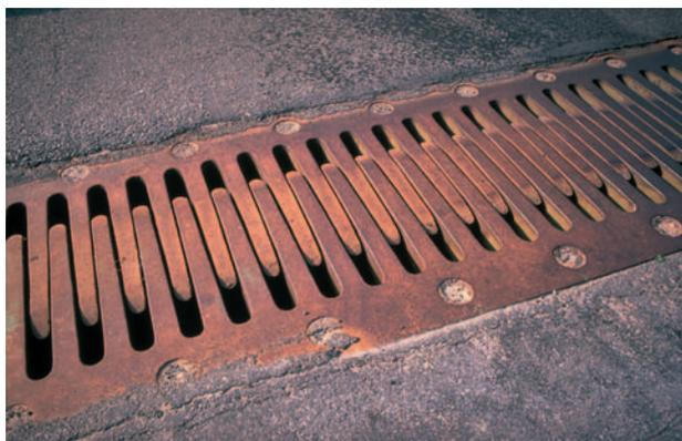
Joints like this one are used in bridges to accommodate thermal expansion. JLM Visuals. Reproduced by permission.
