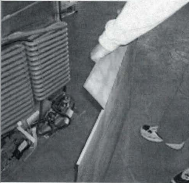
Figure 8-40 Step 3, Installation of Air Channel
