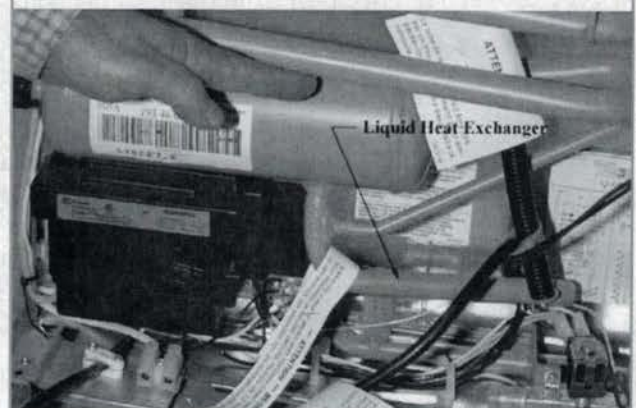
Figure 8-10 Liquid Heat Exchanger
