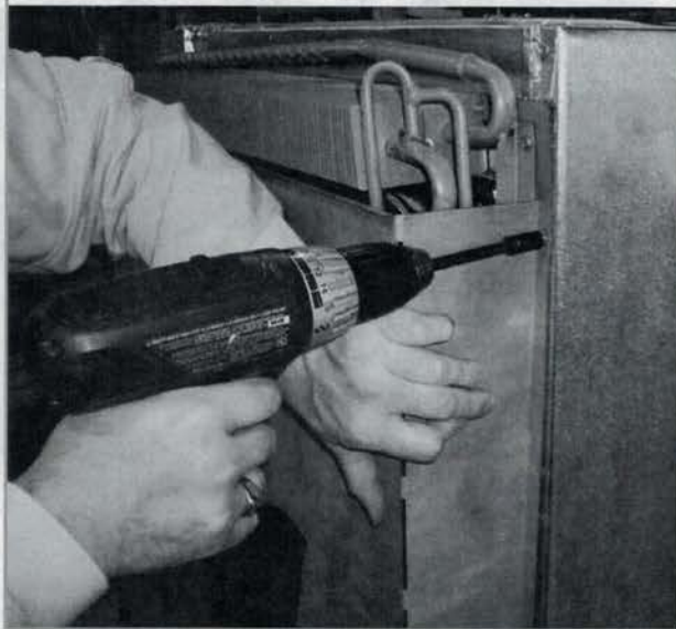
Figure 8-44 Step 7, Installation of Air Channel
