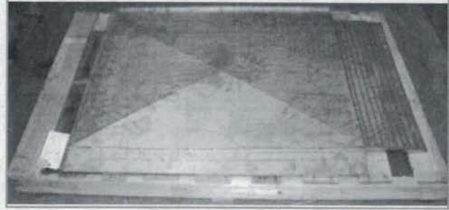
Figure 8-38 Step 1, Installation of Air Channel
