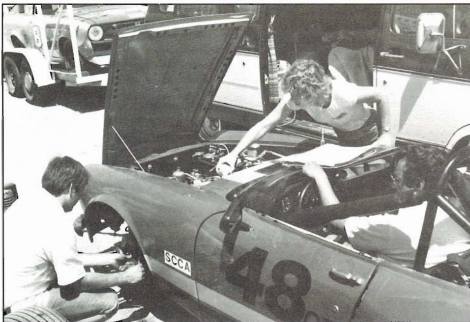
Most racers prefer manual-bleeding method: One person opens and closes bleeders while helper operates brake pedal. Although optional, it's helpful for third person to watch reservoir and add fluid when needed. Method is reliable, but success depends on communication between those doing job.
