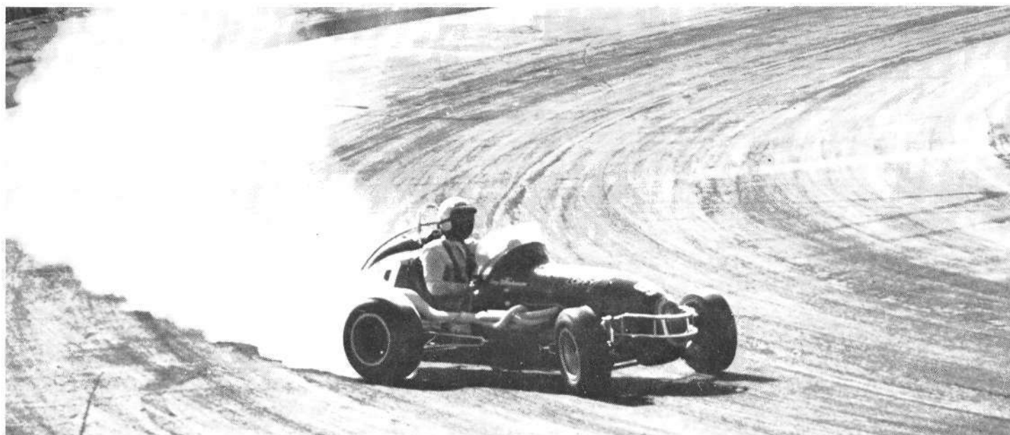
Oval-track racing is all left turns, usually banked, on a dirt or paved surface. The cars are front-engine designs with solid axles in the sprint and midget classes. A midget is shown here in the typical oversteering cornering attitude. Other oval-track cars include stock cars and the rear engine championship cars. (Don Larsen photo)
