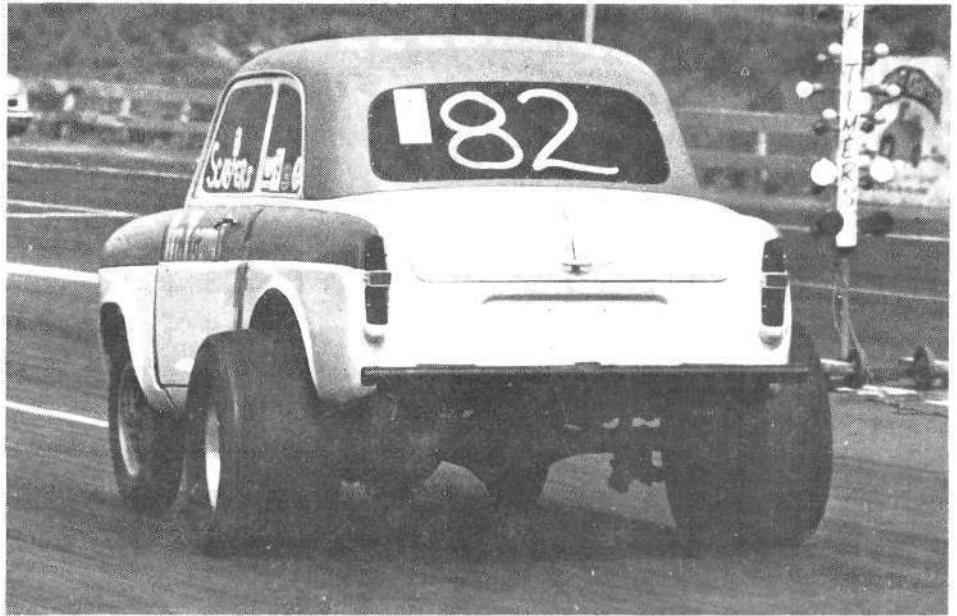
This modified Anglia is equipped with big drag slicks and is raised for better weight transfer. It also has a very heavy rear push bar to move its CG back slightly. This trick is not legal in the stock class.
